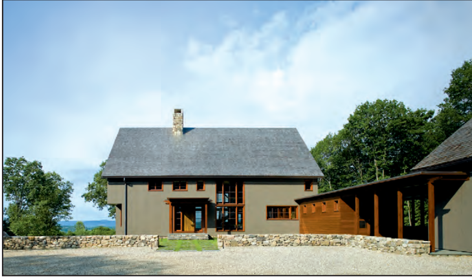
Facing page, top, the West side of a Kent residence designed by Halper Owens Architects LLC of Washington and Greenwich, and bottom, the South side. Clockwise from above, the East side, a fireplace, an interior staircase and the kitchen, all in the same home, whose design won an award from the state chapter of the American Institute of Architects.
